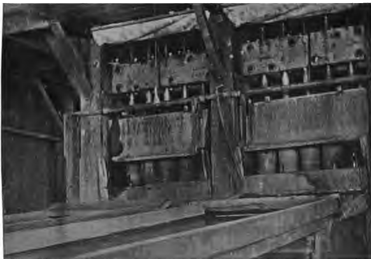
FIG. 103.—THE STAMPS IN A QUARTZ-MILL
